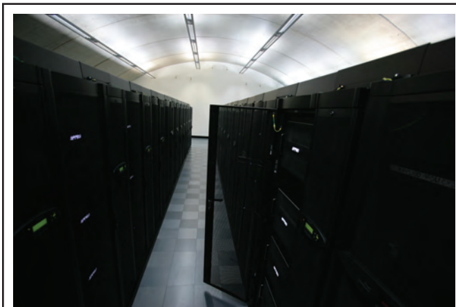
Scalable supercomputing clusters with ultradense CPU/GPU dual-core processors give oil and gas companies high-performance capabilities with up to 1,000 teraflops of compute power at lower cost. Scalable “building block” architectures make it easier and more cost effective for smaller oil and gas companies to adopt HPC technology.
